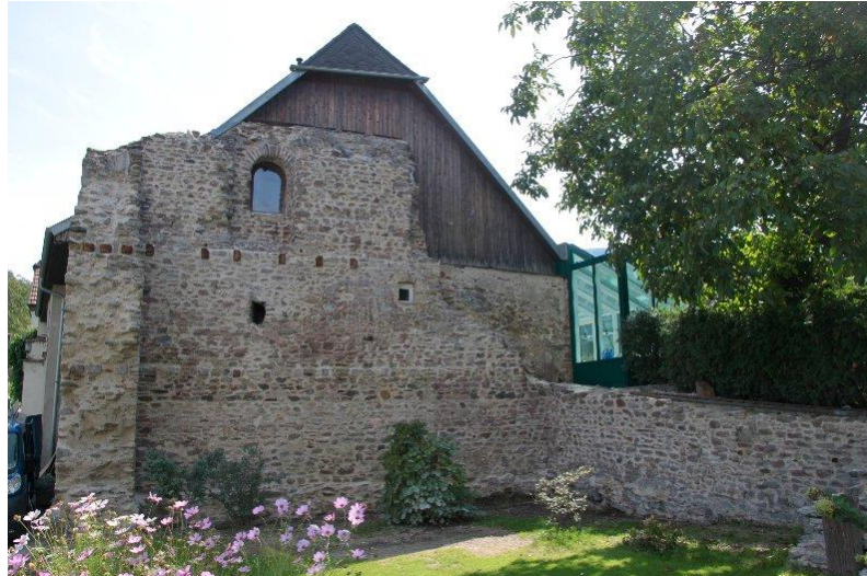
Figure 40: The preserved walls of the burgus at Bacharnsdorf (Lower Austria). The impressive thickness of the walls and their preservation up to the second floor are still visible (© Bundesdenkmalamt, photo: Christoph Tinzl).
