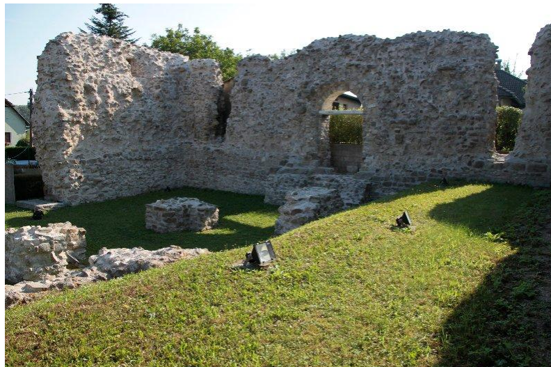
Figure 39: In Mautern (Lower Austria), formerly known as Favianis, the late antique tower buildings are still excellently preserved and open to visitors today (© Bundesdenkmalamt, photo: Christoph Tinzl).
