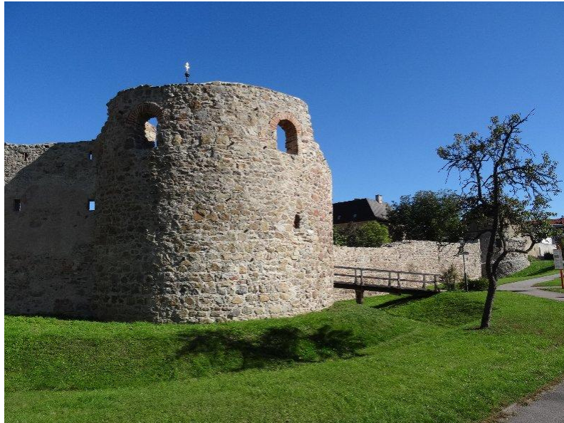
Figure 38: An exceptionally well preserved late antique U-shaped tower in the Mautern fort (© Bundesdenkmalamt, photo: René Ployer).
