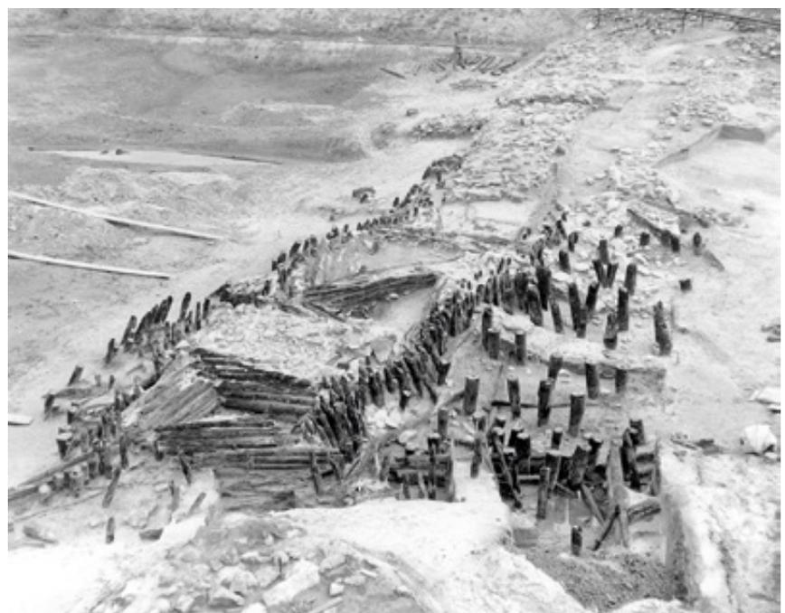
Fig. 44 A barrier at the bottom of the riverbed: a line of wooden caissons filled with stones (Channel 2).
